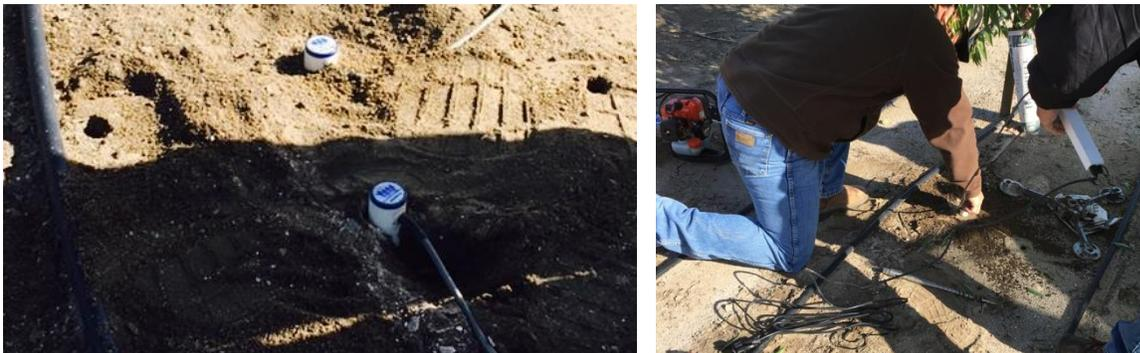
Figure 9: SENTEK soil moisture probe installation
